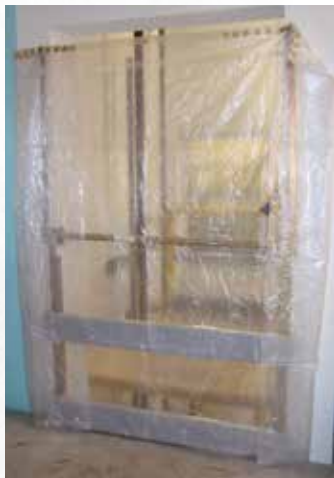
Variant 2: Extensive lift shaft entrance protection
