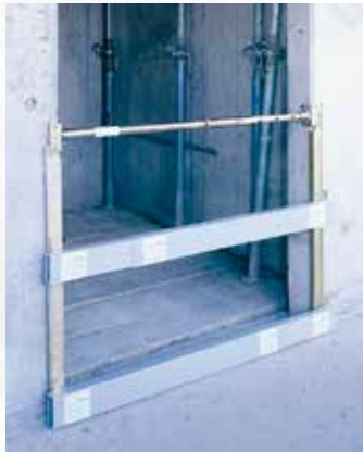
Variant 1: Partial lift shaft entrance protection
